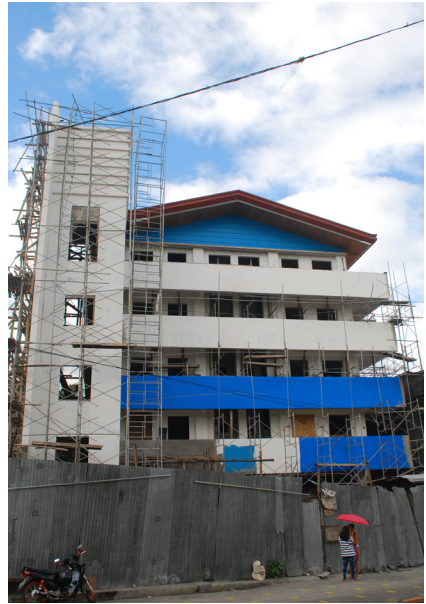
On-going construction of the Cobey Property-Medium Rise Condominium.
