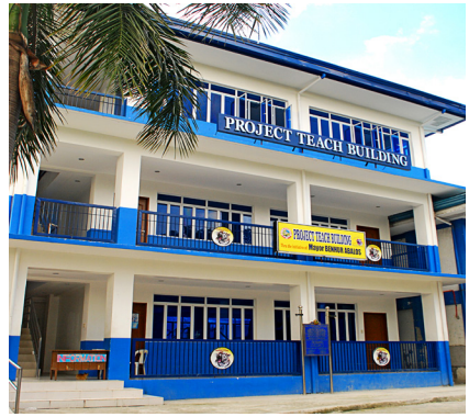
Project TEACH building located at Hardin ng Pag-Asa, Brgy. Addition Hills
